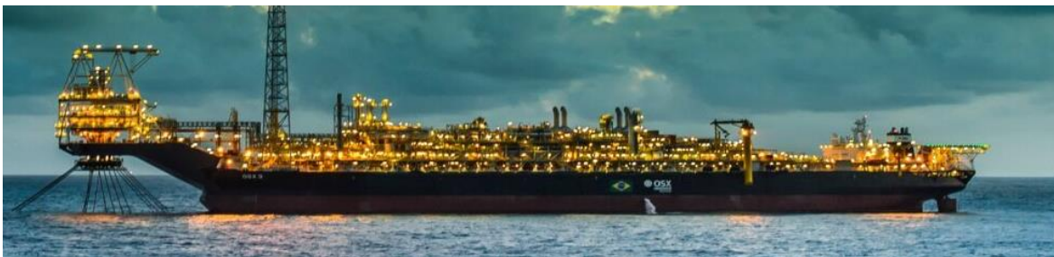
OSX-3 FPSO no Campo TBMT
